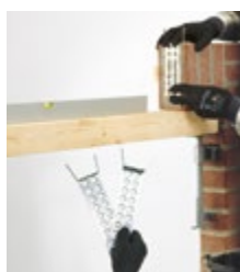
▲ ... on the bricks during bricklaying
