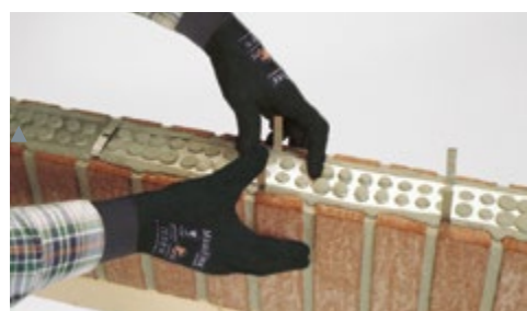
▲ ... and place MOSO® perforated strip between the hangers after completing the Grenadian layer. Then simply bend the perforated strip hangers closed. Finished!
