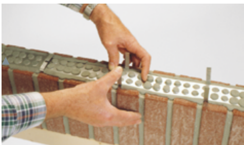
▲ ... and place MOSO® perforated tape between the hangers after completing the Grenadian layer. Then simply bend the perforated tape hangers closed. Finished!
