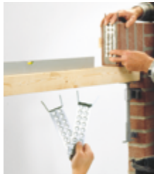
▲ ... on the bricks during bricklaying
