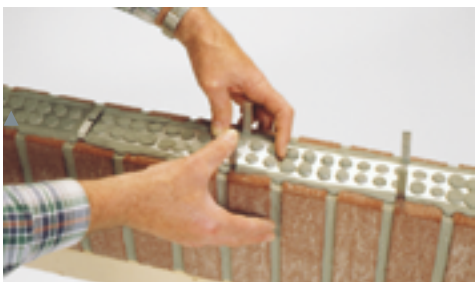
▲ ... and place MOSO® perforated tape between the hangers after completing the Grenadian layer. Then simply bend the perforated tape hangers closed. Finished!
