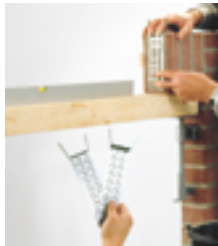
▲ ... on the bricks during bricklaying
