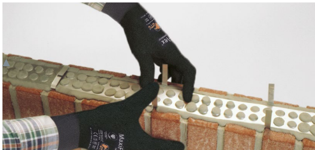
■ ... then place a longitudinal piece of the MOSO® Lochband, press it into the mortar and finally bend the steel tabs over the Lochband. Finished!
