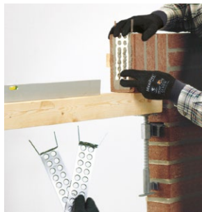
■ ... between bricks for the soldier course lintel
