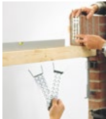
▲ ... on the bricks during bricklaying
